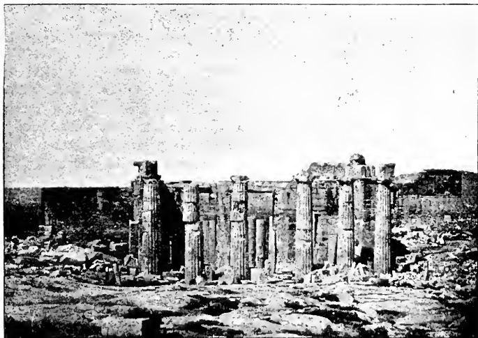
FIG. 7.—VIEW OF PROPYLAEA, SHOWING DOUBLE ANTA.
